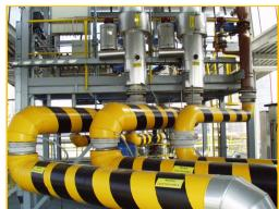
Our On Spot loading facilities to fill rail-bound tankers with liquid products are designed for high filling capacities. Filling pipes of up to DN 300 (NPS 12 inches) provide for loading capacities of up to 1,000  $\rm m^3/h$  (4,400 gallons per minute) per loading point (filling station). Several products can be loaded at one station. To operate a double-track loading facility of 20,000 tons per day, only one or two operators are needed in the control station and another one or two helpers.
